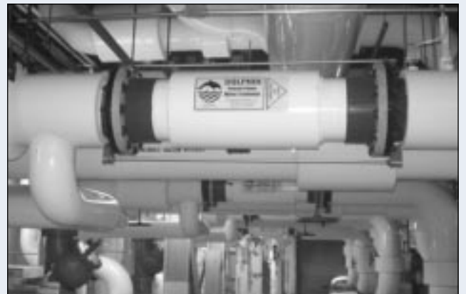
Dolphin System Installation at the West Virginia Capitol.
