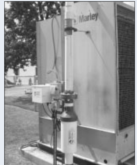
Dolphin Installation at SMMC.
