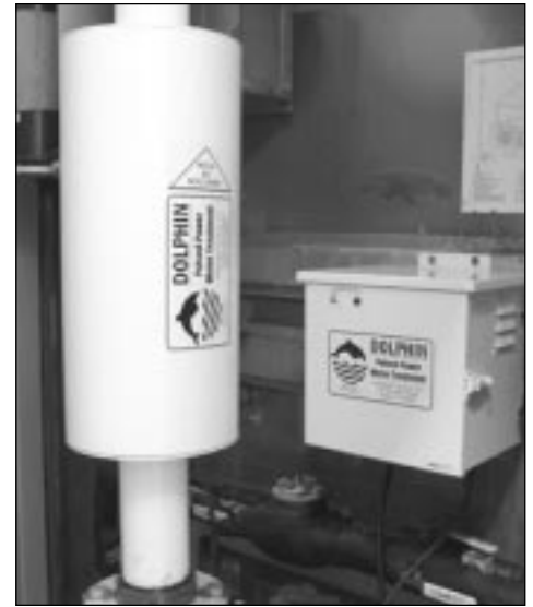
Dolphin Installation on Mammoth Unit.
