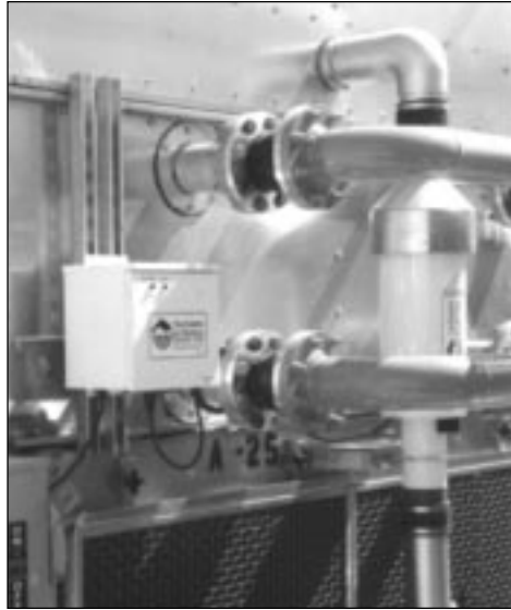
Red Bluff: One of 16 Dolphin Units.
