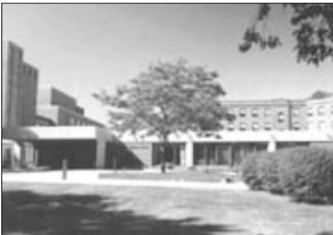
Lawrence & Memorial Hospital
