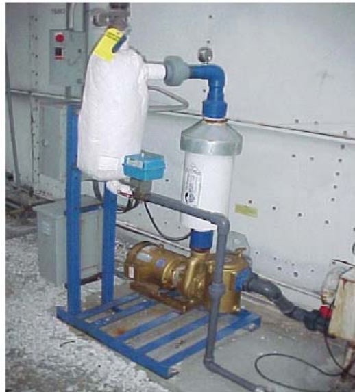
Figure 2. 3" PP with Insulated Cyclonic Separator
