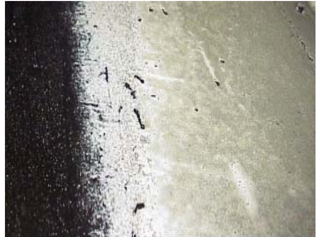
Figure 14. Chemical Tower – Scale on Sidewall
